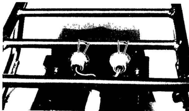
4. Turn the bulb counterclockwise and remove the defective bulb.
